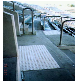
Figure 4: The tactile marking (mat) is a haptic focal point to draw attention to possible danger.
